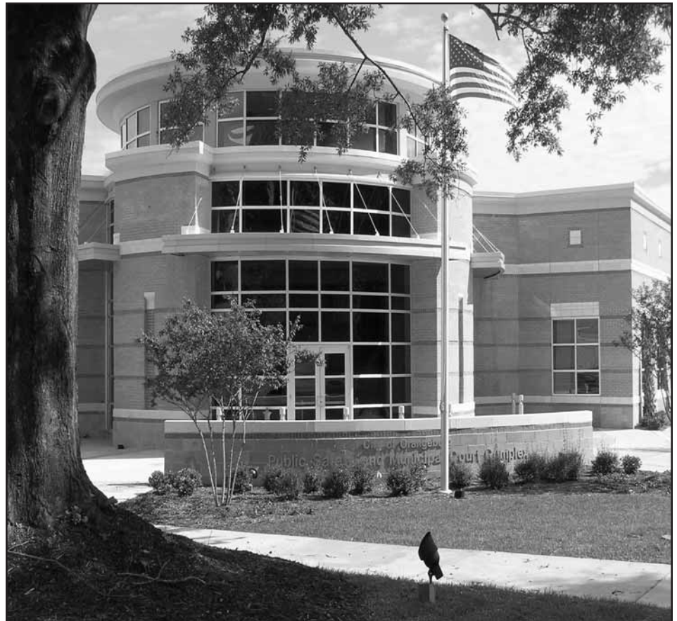
Outstanding New Construction Project - Orangeburg
